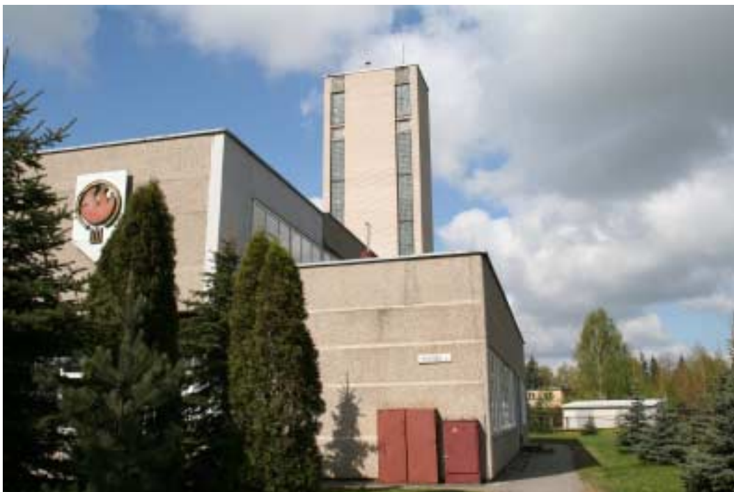
Fig 4. GPS antenna on the roof of fire station tower
